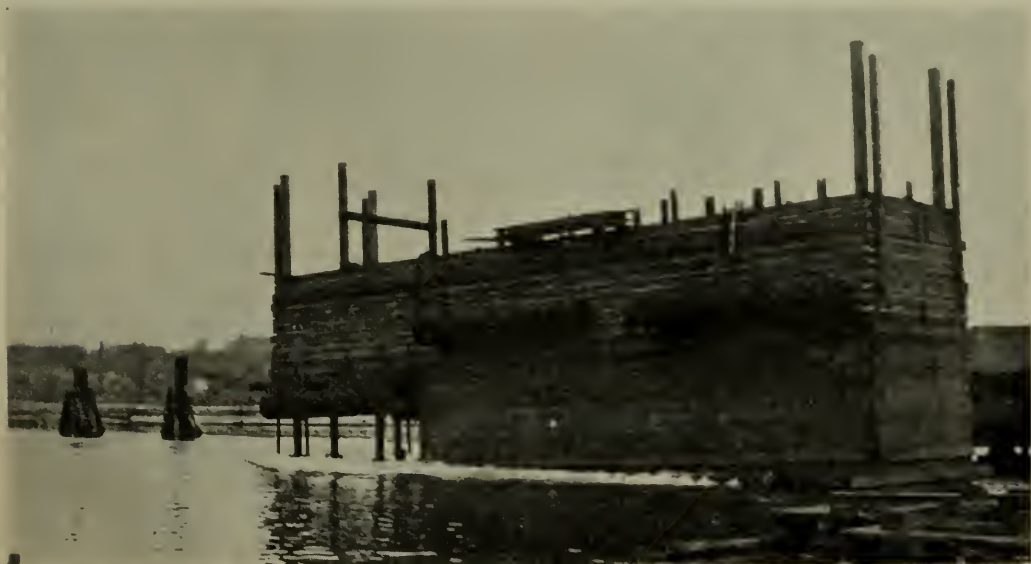
FIG. 5. REST PIER CAISSON BEING LAUNCHED.
